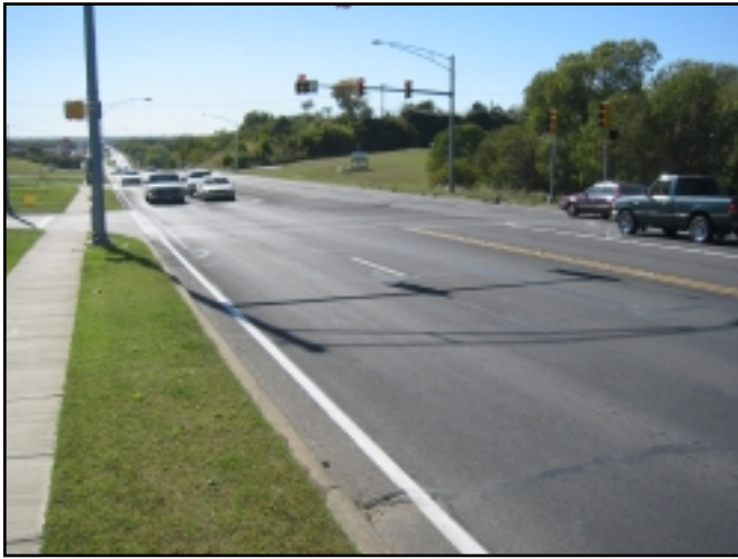
State Highway 183, N. W. Fort Worth, Tx, 19 year old ESCS overlay, since 1985 over jointed concrete.
